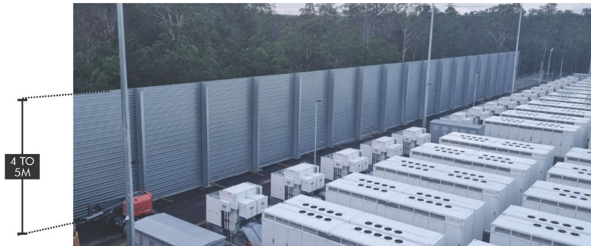
Figure 11 – Example of a radiant heat wall between BESS units and a forested area.
